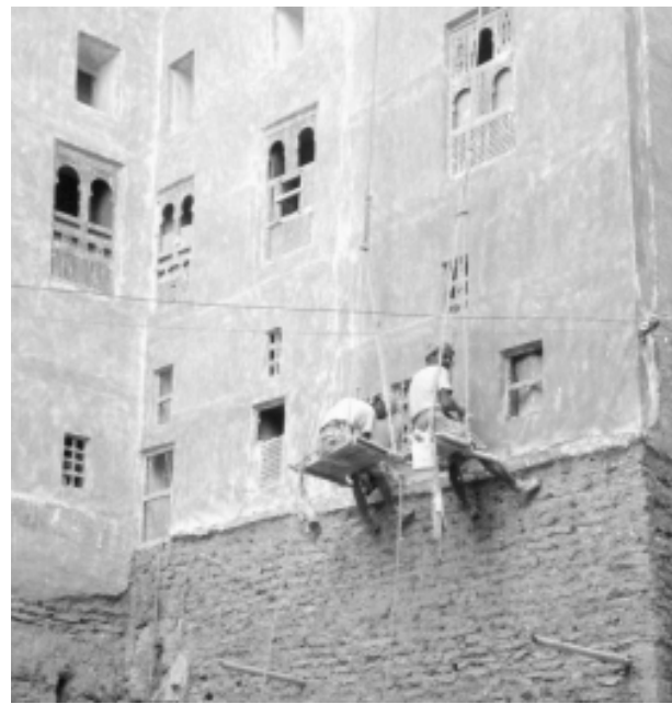
Workers in Shibam maintain the facade. Photograph: Maria deJ. Ellis 1998.
